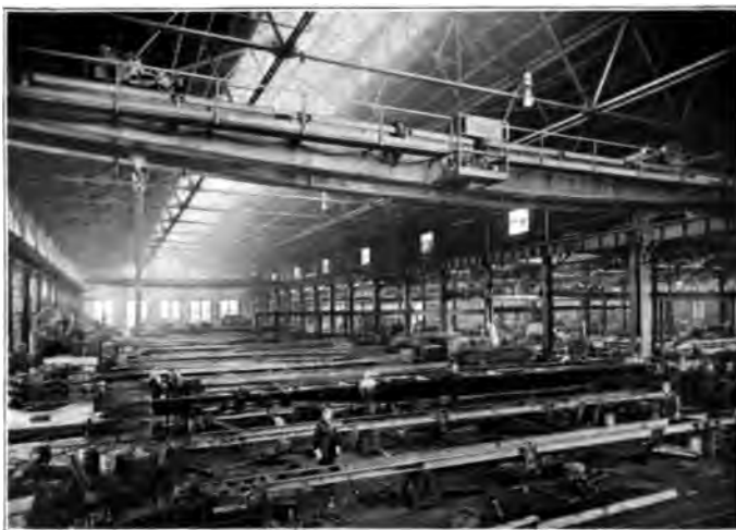
Fitting up the steel car underframe. Steel Erecting Shops
